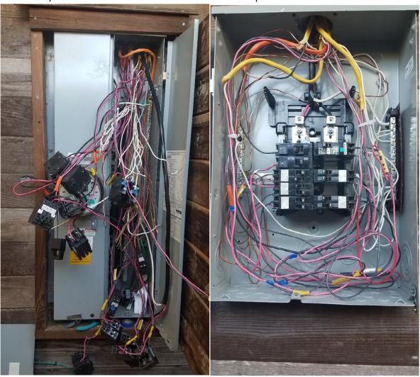
Breaker boxes are set for 240vac, two hots, a common and ground bar. One hot serves half the breaker spaces and the other hot serves the other half. I wanted all the critical breakers on one
